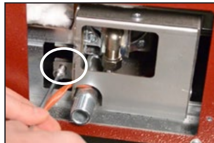
5 - Tighten the burner fixing screws.
